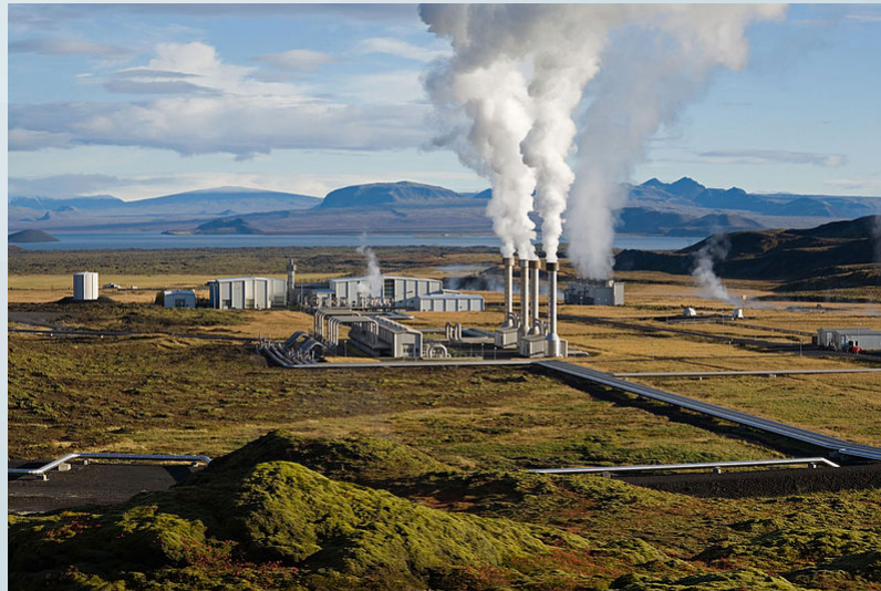
Nesjavellir Geothermal Power Station in Iceland
